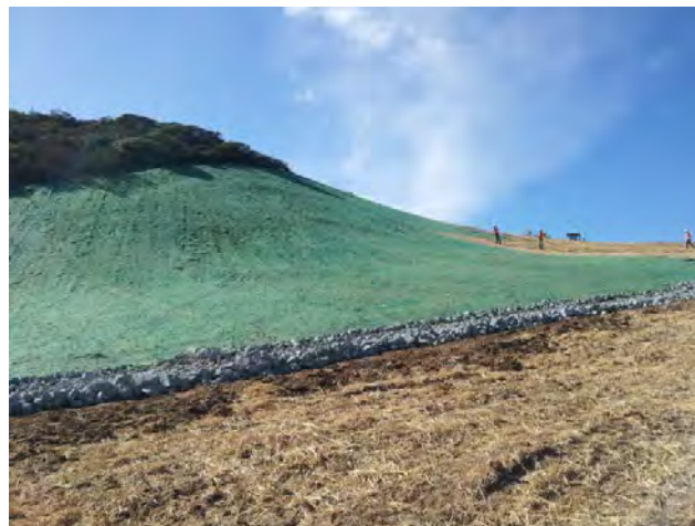
Upper Coir Fabric slope with hydromulch.
