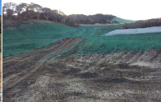
Lower-site post hydro-mulching
