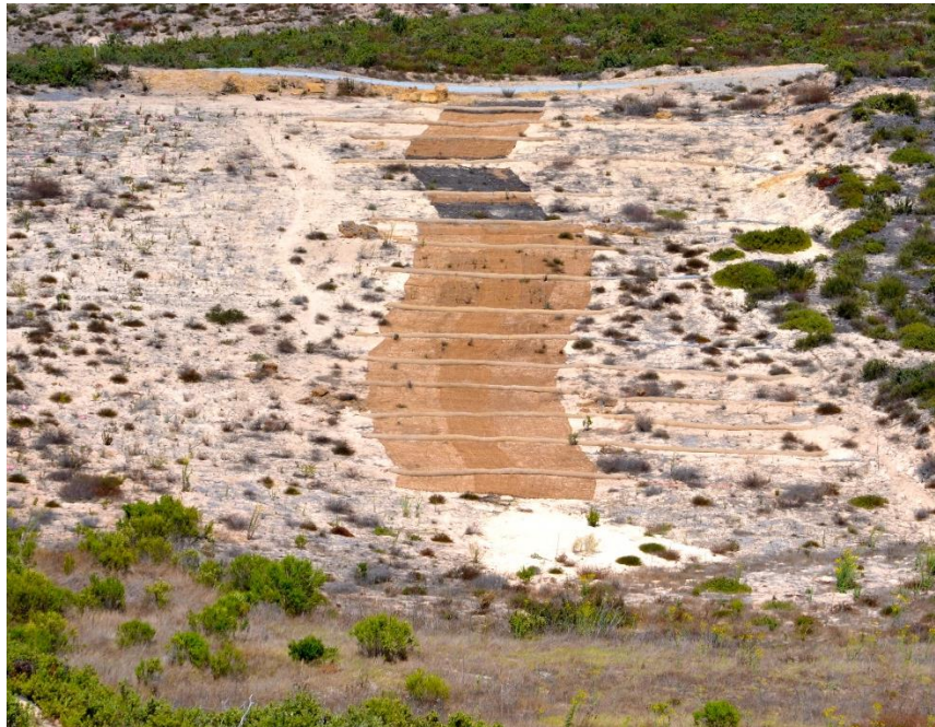
Figure 1 HA 28 post erosion control repairs.
