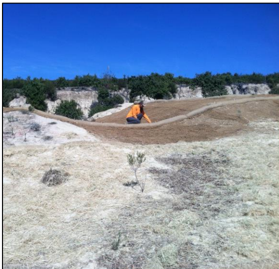
Photos 3: After erosion control repairs at HA 27A.
