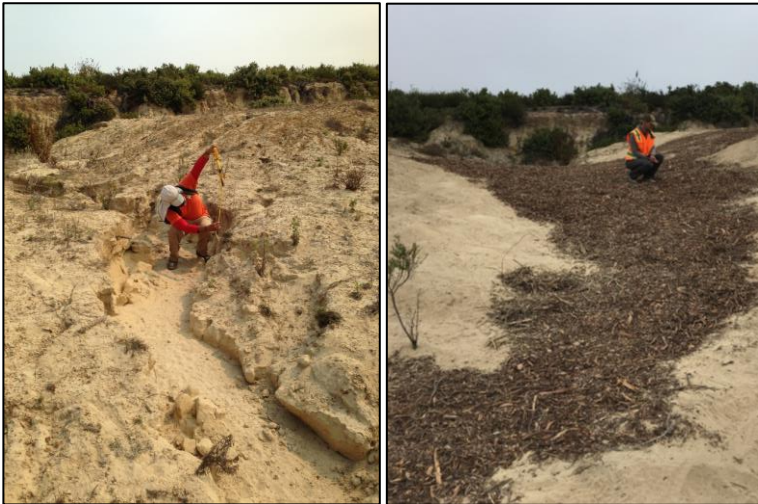
Photos 1 & 2: Before and during erosion control repairs at HA 27A.
