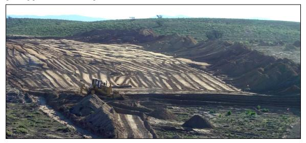
Photograph 7-1 — Bulldozing the top 2 feet of soil into the center of Range 45 allowed sifting the stockpile to remove MEC and spoils from the soil.
