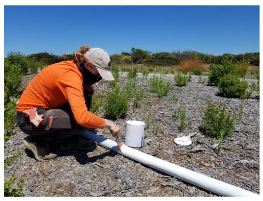
Photo 16: Burleson biologist painting PVC to protect lines from sun damage
