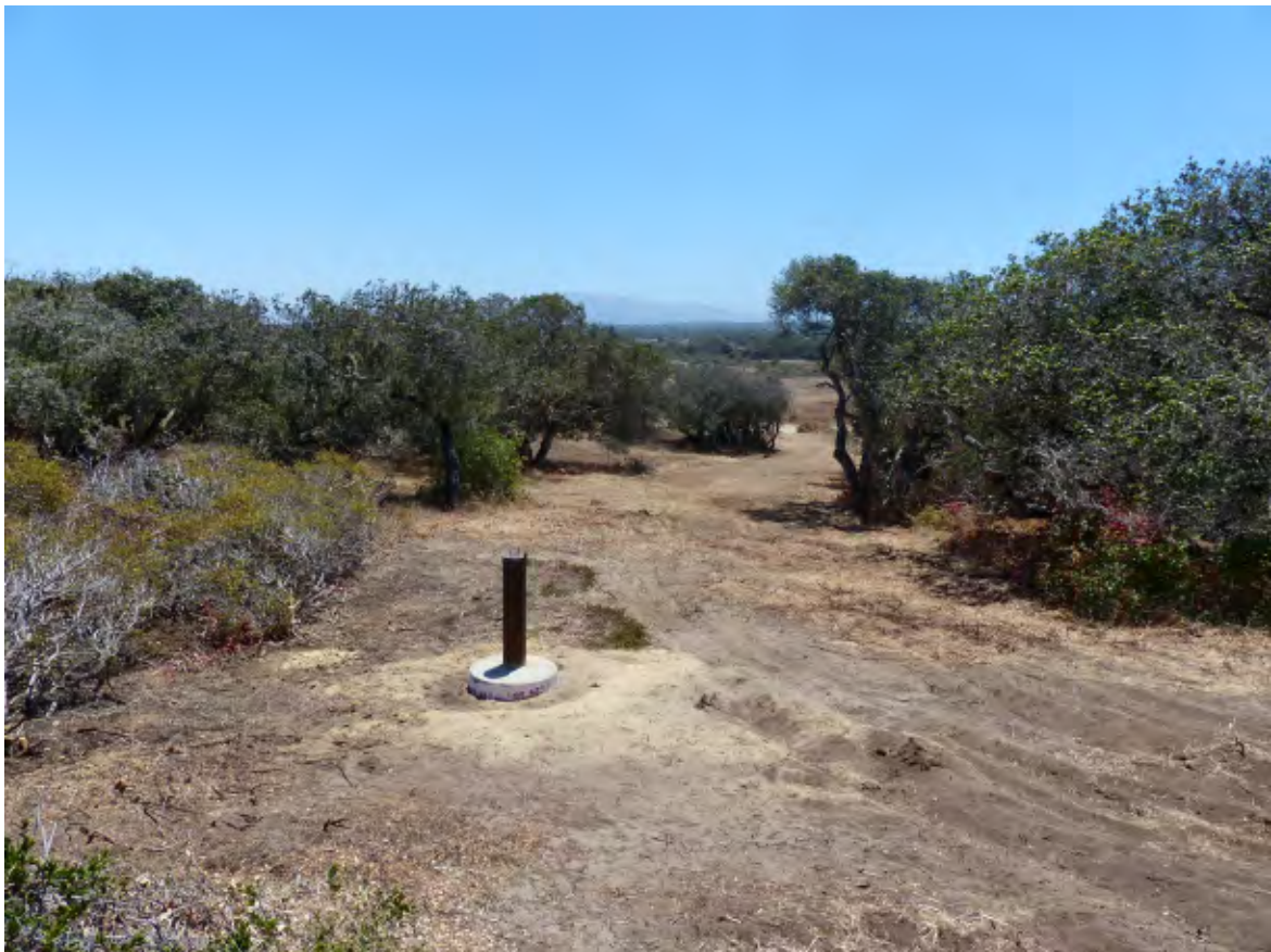
Photo 8. Well MW-BW-88-A facing southeast, after installation.
