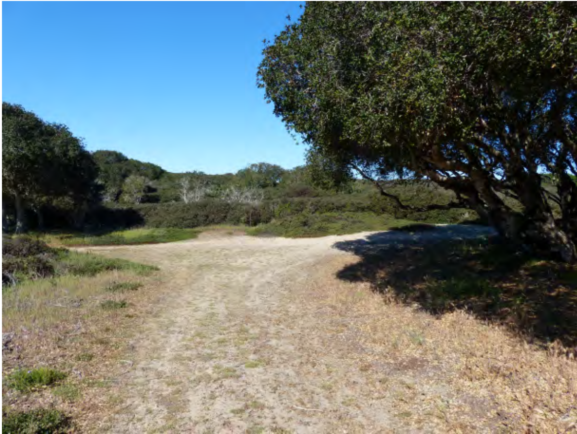
Photo 11. Well installation location MW-BW-89-A facing west, before installation.
