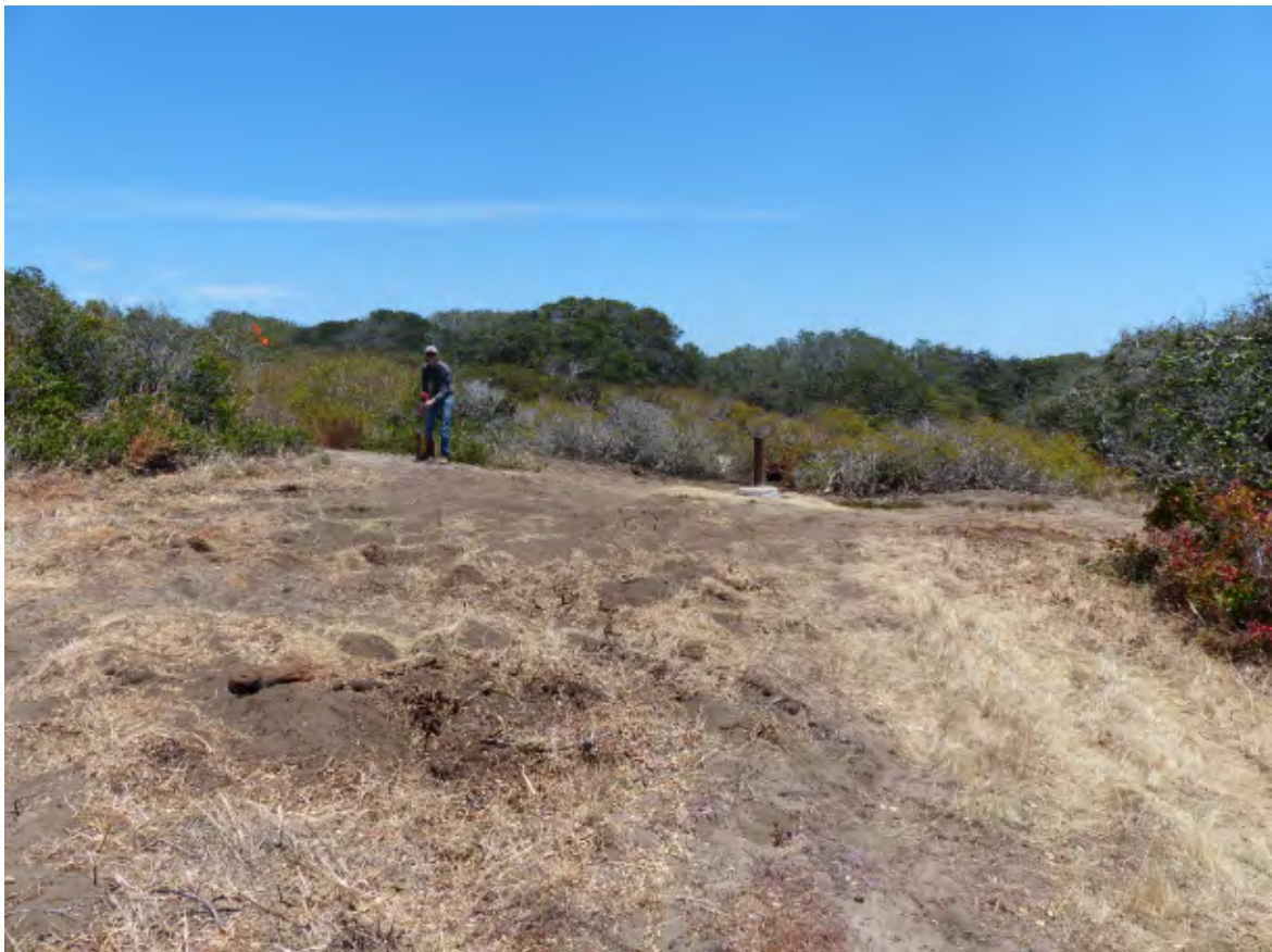
Photo 10. Well MW-BW-88-A facing northeast, after installation.
